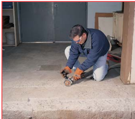
2. Joint and crack are squared-off and opened up.
