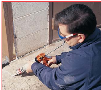
Urethane Sealant being used to seal a crack.
