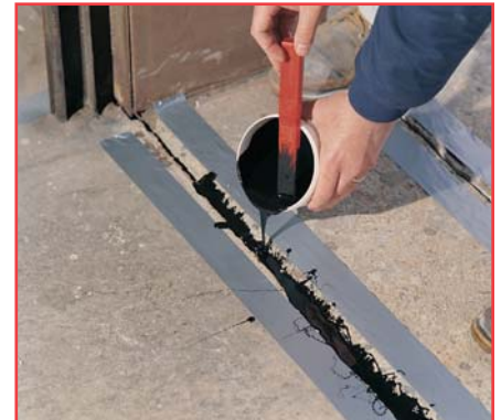
3. Area is taped off and product is poured into joint.
