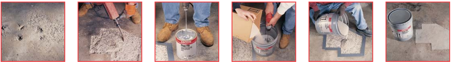
For repairs using Floor Fill, simply square off the repair area and chisel out the loose and damaged area; pre-mix the resin; while mixing, add the aggregate; pour into repair area.
